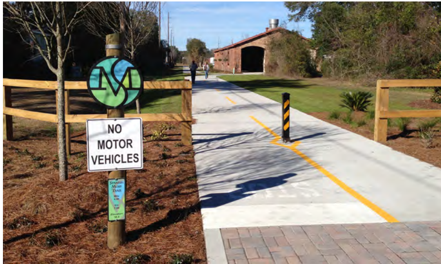
An intersection example at Spanish Moss Trail, Beaufort, South Carolina
