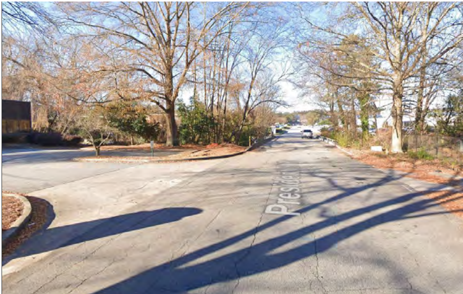
Existing conditions of Presidential Drive, facing west. A proposed at-grade crossing will connect the trail to the future redevelopment of the Clyde Industries parcels.
