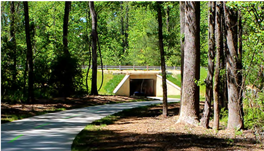
Box culvert structure allows the trail to pass under a roadway where existing road bridge does not exist.
