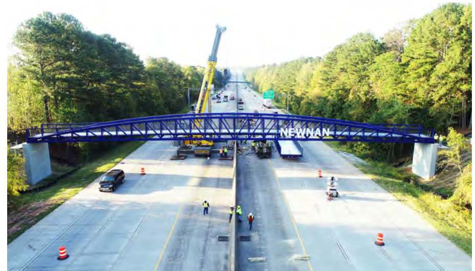
Example of a prefabricated trail bridge over I-85 in Newnan, GA
